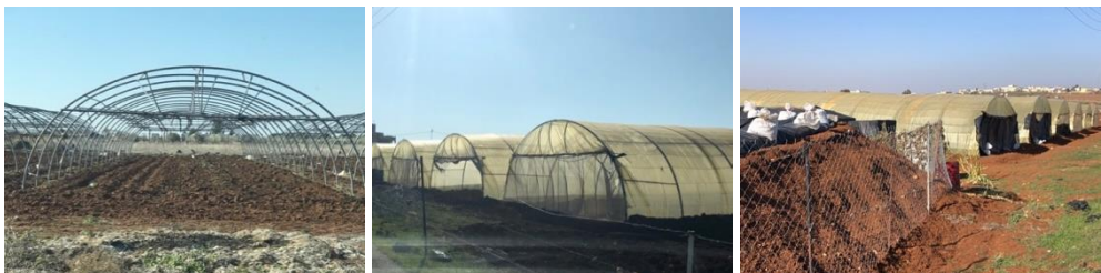
Figures 3, 4 & 5: Construction of 'green houses' at planting time - during the growing season with rainwater storage
