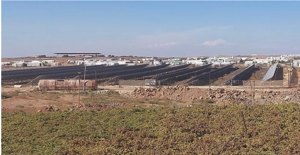
Figure 11: Solar systems on the farm
